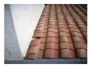
We observed roof tile(s) that are cut so that the material under the tile is exposed. Exposure to the elements can damage the material under the tile and cause roof leaks. We recommend that a qualified roofing contractor replace all improperly cut tiles. The tile(s) requiring attention include: several tiles at roof hips.
