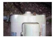
We observed that the pool timer inner cover is absent and that the outer cover is damaged. This is an electrical shock safety hazard. We recommend replacement of the timer box by a qualified technician.
