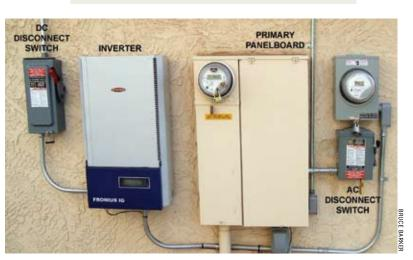
These are typical solar PV system components.
