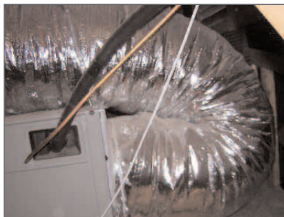
Radius of bend less than one-duct diameter
