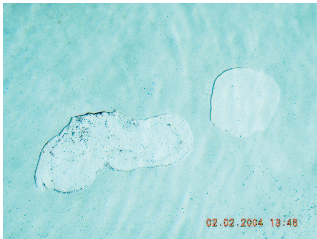
The deteriorated interior surface of a pool in need of resurfacing
