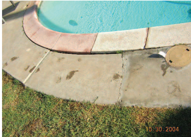
A cracked and displaced pool deck in need of repair
