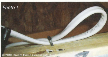
An example of a tight radius bend.
