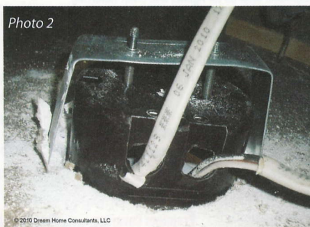
An example of how not to run cable into a box.
