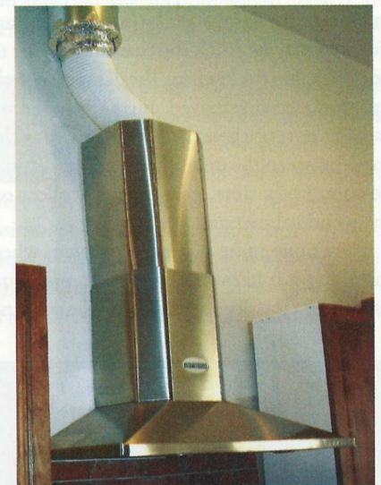
Photo 2: Plastic corrugated exhaust duct really is a fire hazard.
