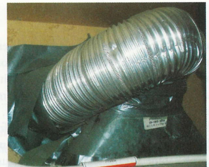
Photo 1: Metal corrugated exhaust duct is a fire hazard.
