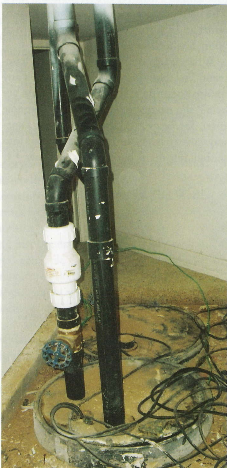
Photo 2: Sewage ejector with gate valve, check valve and a vent.
