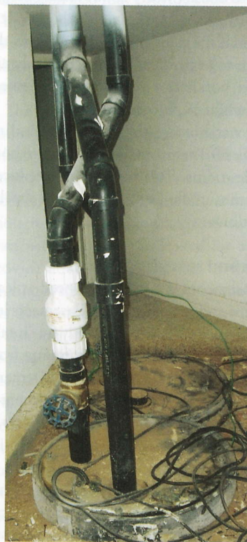
Photo 1: Sewage ejector with gate valve, check valve and a vent.
