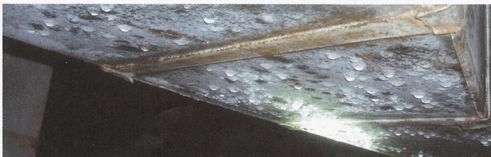
A similar effect can occur in exterior wall cavities, especially around penetrations such as electrical boxes. Negative pressure inside can suck air and water vapor from outside into the cavity. Positive pressure inside can force air and water vapor from inside into the cavity. If enough water vapor condenses in the wall and doesn't dry, hidden damage and mold can occur.
