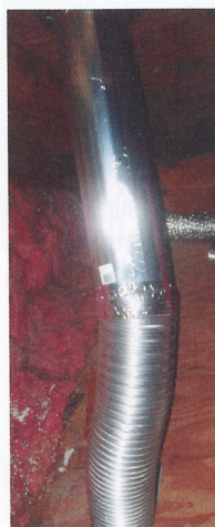
Photo 2. Flexible vent improperly penetrates a ceiling and has been improperly modified. Photo 3. Way too many bends!
