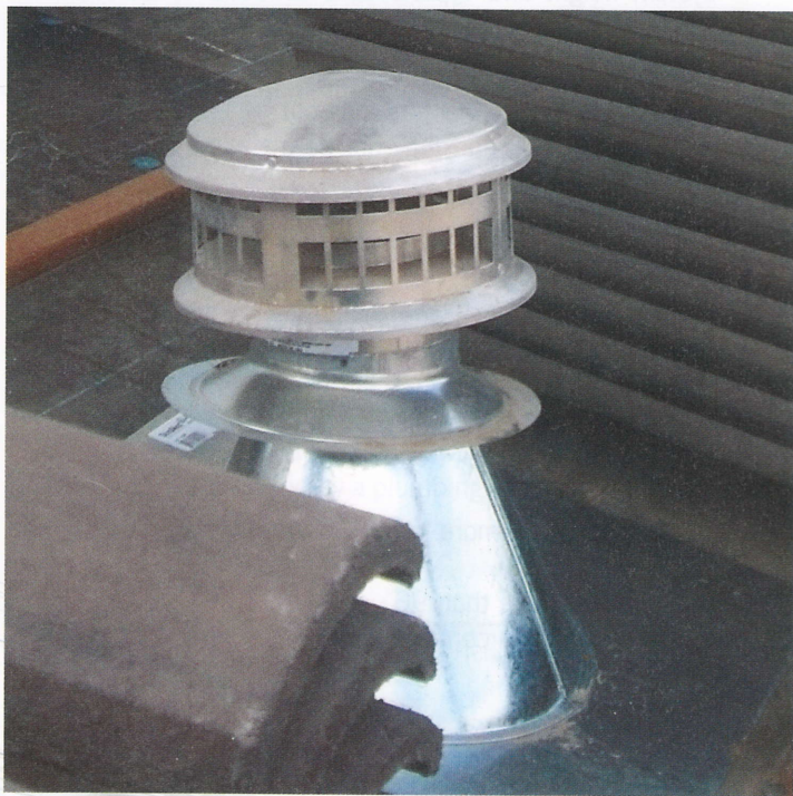
Photo 4. Vent is too close to the roof, too close to the sidewall and too close to the window.
