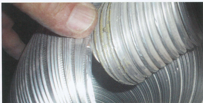
Photo 5. The flex duct from the fan is bad enough, but to air couple it to a bath duct?
