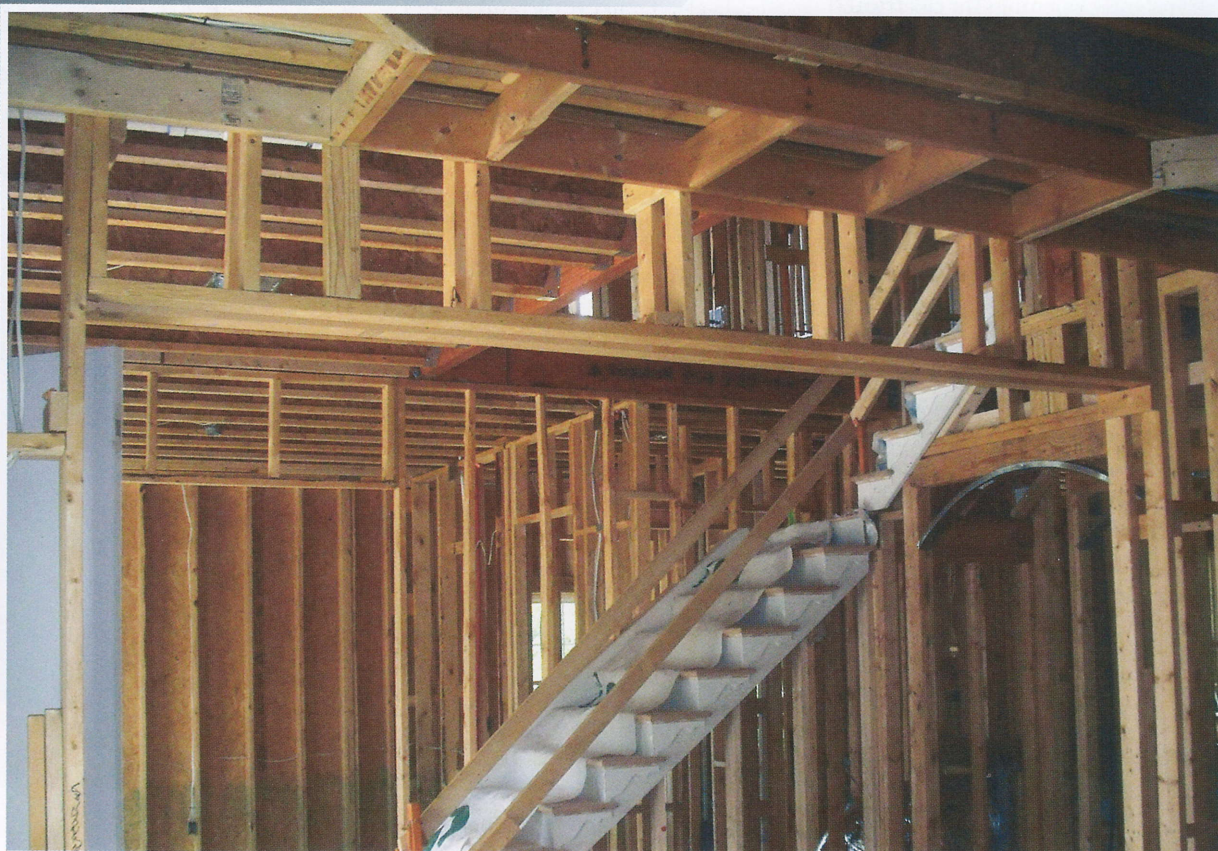
Photo 4. This double-stud header is longer than 10 feet and should be fireblocked near the center.
