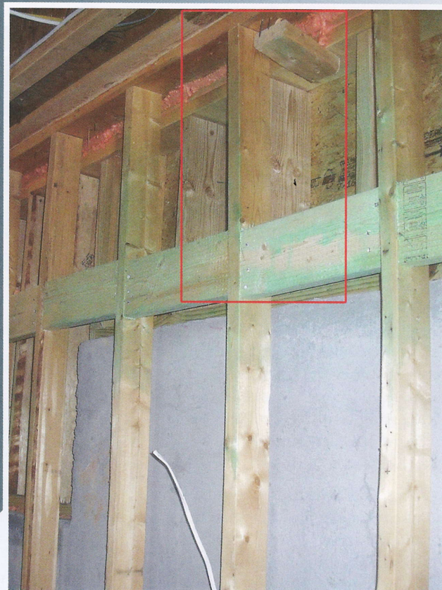
Photo 3. Fireblock double walls every 10 feet both, as shown in the red box, and also along the foundation.
