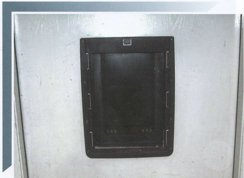
Photo 7. No pet doors allowed between the house and the garage.
