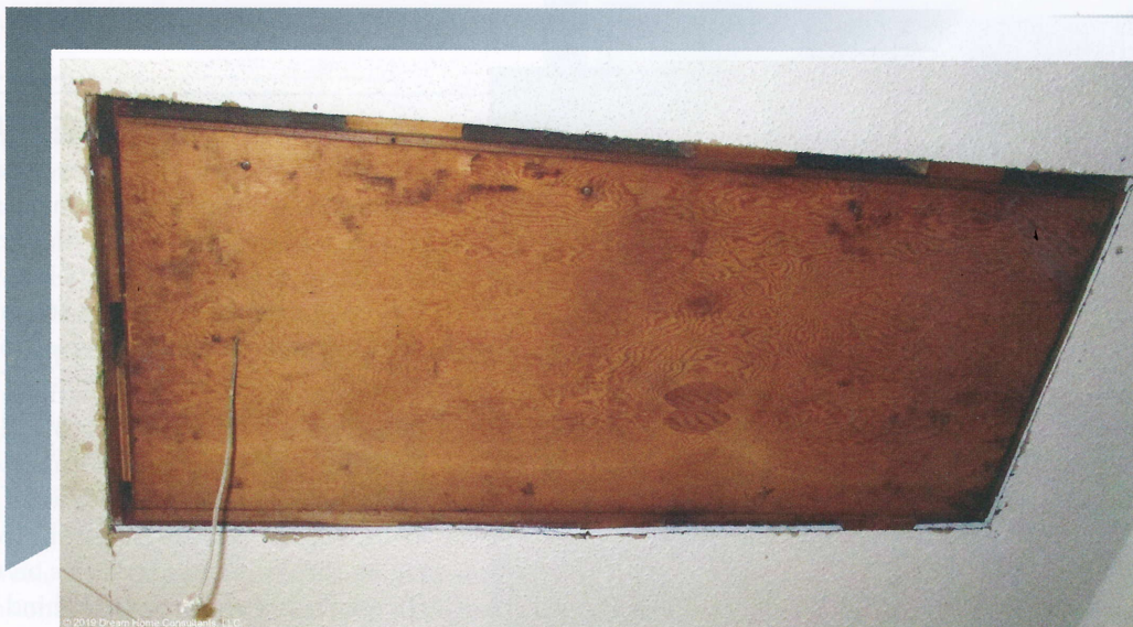
Photo 8. Pull-down stairs are almost always wrong in a garage.
