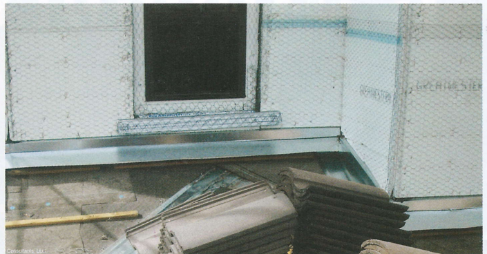
Photo 4 XPS insulation board is often used as sheathing under one-coat stucco. It will be covered on both sides, so there's no ignition risk.
