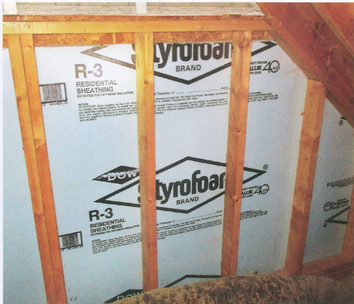
Photo 3 This Extruded Polystyrene Foam (EPS) insulation board should be covered in an attic. It says so right on the board.
