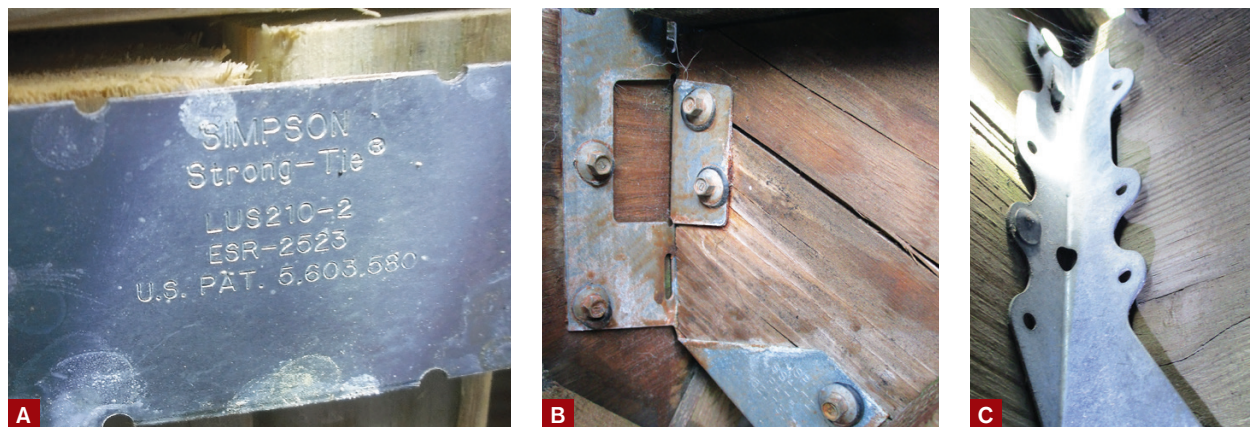
Figure 3. White rust is already forming on this joist hanger, which is only approved for interior use (A). Metal-roofing screws aren't approved joist-hanger fasteners (B), nor are roofing nails (C); all of the holes in metal hardware should be filled with approved hanger nails or structural screws, and the hanger flanges should fit snugly against the joist (D). Metal hardware shouldn't be field-modified; with its seat removed, this hanger provides minimal joist support (E).
